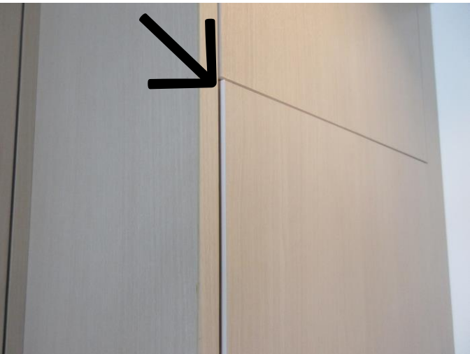
The door of fridge and freezer was not even with the left cabinet panel. It is likely to be cosmetic issue.
