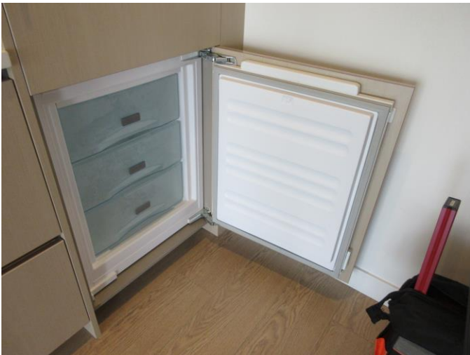
The door of fridge and freezer was not even with the left cabinet panel. It is likely to be cosmetic issue.
