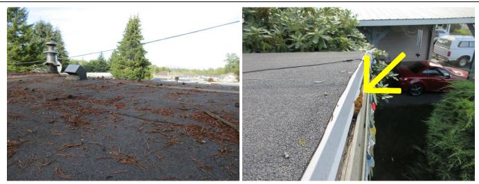
The tree leaves covered the roof surface of the house. Debris and tree leave cleaning around the roof is recommended.
