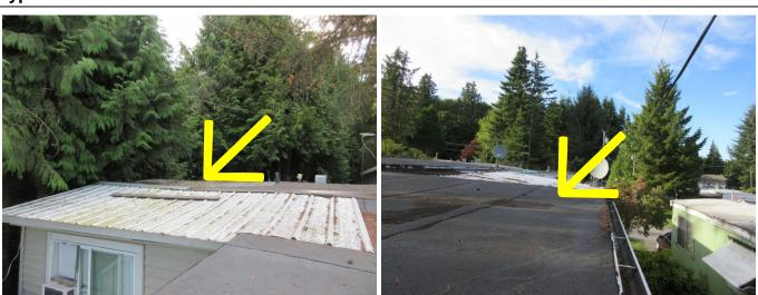
A significant sagging and wavy surface was noted on the roof. The sagging and wavy surface of the roof is the significant deficiency and indicate the potential of the moisture entering to the house. The sagging needs to be fixed, and maintained by the qualified contractor as recommended.
