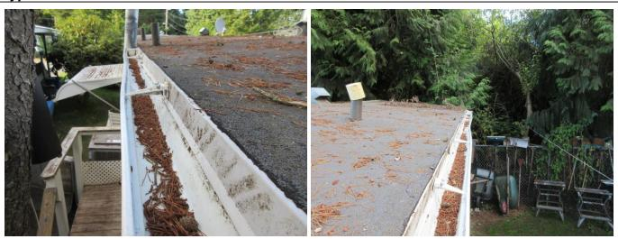
The debris and tree leaves were noted inside of the roof gutter. I recommend clean the gutter to prevent any water leakage to the house. Gutters that drain poorly or clogged can lead to many costly roof edge. It can also cause gutters to pull loose and lead to possible water intrusion.
