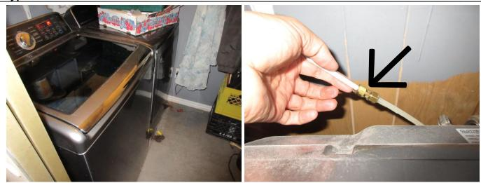
The washing machine and dryer were tested in the laundry room. There was no water leakage for washing machine. The washer and dryer were both functioning at the time of this home inspection. The supply water for the fridge had water leakage in the back of washing machine. Fixing the water leakage is recommended.
