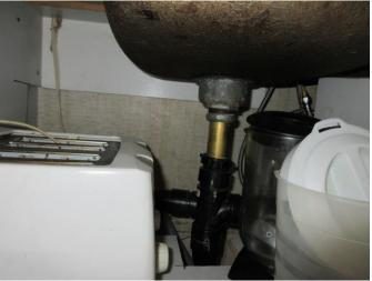
The water leakage was noted under the kitchen sink sewage pipe. I recommend fixing the water leakage.
