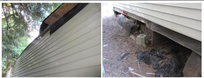
The house exterior wall had vinyl siding. The vinyl wall covering was missed at south and west side of house. Installing the vinyl panel to block entering rodents is recommended.
