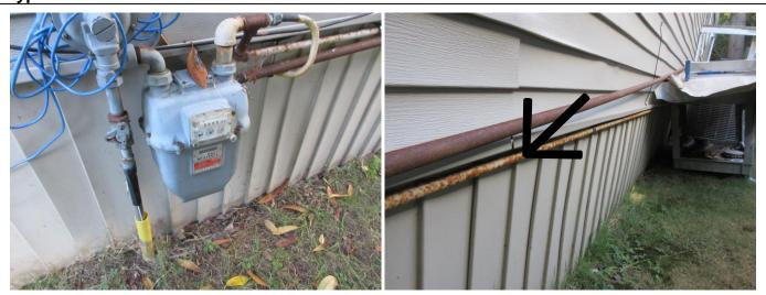
The natural gas meter was located on the west side of the house. The natural gas meter pipe was rusted. I recommend fixing and repainting the gas meter pipe.
