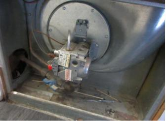
The furnace was a mid-efficiency type with input 40000 BTU. The furnace manufactured in dated 2003. The furnace life expectancy is 15-20 years. The Furnace is 19 years old and has passed its expected service life. Expect to replace the furnace. However, the furnace was functional with no deficiency at the time of this inspection.
