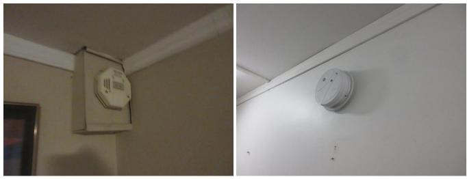
The smoke detectors and monoxide carbon detector were observed in the house. The smoke detector needs to be replaced after 10 years and the battery needs to be checked annually. Replacing the smoke detector when moving into a new residence is recommended.
