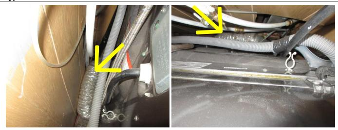
The dryer had foil duct which is not recommended for the dryer. This a safety concern. It is a potential fire hazard. The hard metal or aluminume type duct only is accepted and recommended for dryer. I recommend installing the hard metal or aluminum duct for the dryer.
