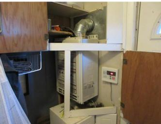
The tank less water heater was manufactured dated 2019. The thankless water tank life expectancy is more than 20 years. It has no leaks and is functioning well at the time of this home inspection.
