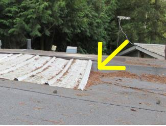
The combination of the torch-on (asphalt rolling) and aluminum sheet were the coverage of roof. The cavity was noted on the connection point of asphalt rolling and aluminum sheet. Any cavity had the potential of the moisture entering to the house. It appears the best tradesman practice was not applied to the roof covering.
