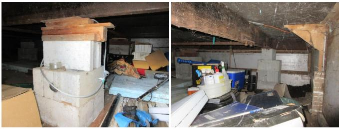
The mobile house had base concrete foundation. The mobile house was not fasten to the ground. This is significant structure deficiency. I recommend contact a qualified contractor for further evaluation and fixing the issue.
