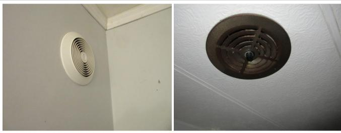
There were electrical exhaust fans in the bathroom and the washroom of the house. The exhaust fan in the master washroom and main bathroom were functional with no deficiency at the time of this home inspection.
