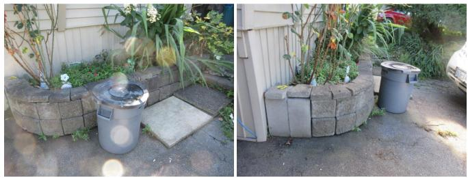
The house had masonry stone retaining wall on the north side of the house. The uneven surfaces and moving blocks were founded on the retaining wall. Fixing the retaining wall is recommended.
