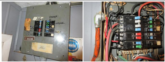
The electrical panel was 100 Amp and was located in laundry room and professionally was installed. The wire type of the house was copper. It shows no burnt, damaged, or corroded wires. Appropriate circuit breakers and sized wires were used for specific circuits (i.e. 40 amp for the range, 30 amp for the dryer, and 15 amp for general circuitry). The incomplete breaker label was noted. Sticking the full breaker label is recommended.
