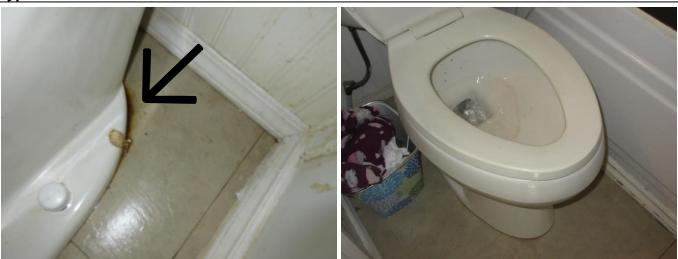
The water leakage was observed at the back of the toilet in the bathroom of the house. I recommend fixing the water leakage by a qualified contractor.
