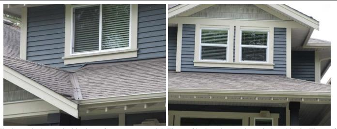
The house had asphalt shingle roof coverage material. The roof had no damaged or missing shingle. The roof coverage was functioning well at the time of this inspection. The roof coverage with proper care they should serve the house for many years. Typically, asphalt shingle normal service life is 15-20 years. The asphalt shingle seems to be in the second half of its useful life.
