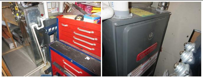
The house had combination of furnace and A/C. The furnace manufactured in dated 2012. The Furnace is 12 years old. The furnace life expectancy is 15-20 years. The furnace was functional with no deficiency at the time of this inspection.
