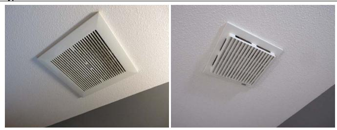
There were electrical exhaust fans in the bathroom at the basement and seconed floor of the house. The exhaust fan in the master bathroom and main bathroom were functional with no deficiency at the time of this home inspection. The main bathroom electrical exhaust fans grill was dirty and clogged with dust at the second floor of the house. I recommend cleaning the grill of the fan for better functionality.
