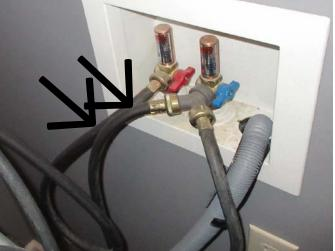
The rubber hose was used for the supply water of washing machine. The water pressure can expand the rubber hose in the long time. The expanded hose may cause the hose has water leakage. I recommend changing the rubber hose type with the (Braided Metal) flexible tap connector type.
