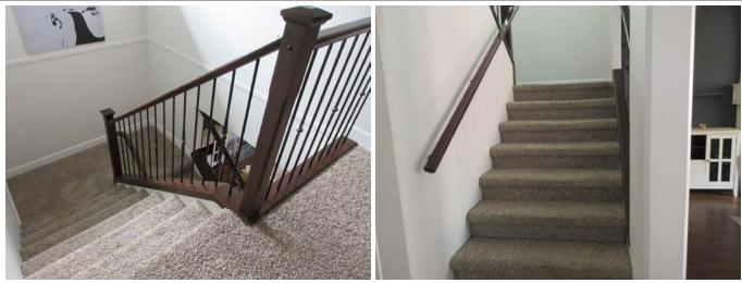
The interior stair was covered by carpet. The stair was functional and the handrail was installed properly with no deficiency at the time of this home inspection.
