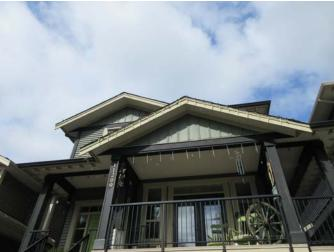
The house had wood fascia and aluminum soffits type. The fascia and soffits seems to functioning with no deficiency at the time of this home inspection.
