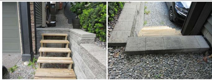
There was no the handrail and guard for stair at the north side of the house. This a safety concern. I recommend instaling the handrail and guard to make it safe.
