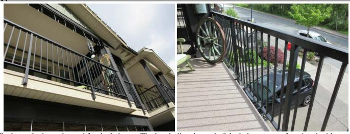
The house had metal guard for the balcony. The handrail and guard of the balcony were functional with no deficiency at the time of this home inspection.
