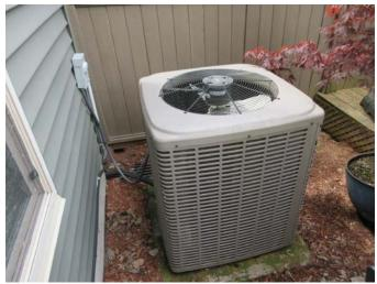
The house had combination of furnace and A/C. The cool mode was not tested due to exterior temperature being below 18°C degrees. Running the unit in this condition can damage the compressor. If concerned about the condition of the unit, request bill of service from homeowner. Both the furnace and AC should be serviced annually.
