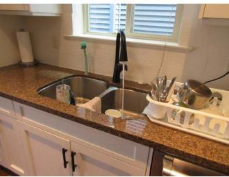
The kitchen of the house had steel sink type. The faucets and sink were functioning with no leaks at the time of this home inspection. The water fixture seem to be in satisfactory condition. The water pressure and drainage seem adequate for the kitchen sink.
