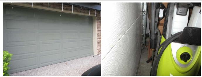
The garage door was functioning and mechanically smooth. The sensors were in place for the garage door and reversed the door at the time of this home inspection.
