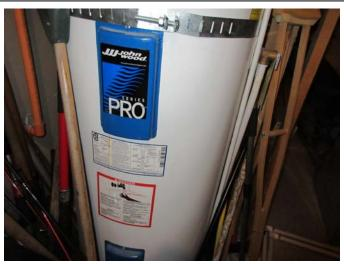
The hot water tank was manufactured dated Oct 2012. The hot water tank is 12 years old. The water tank life expectancy is 7-12 years. The hot water tank useful life was over and need to be replaced with the brand new. It had no leaks and was functioning well at the time of this home inspection.
