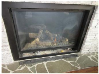
The house had gas fireplace type. There was no protective safety screen / glass in front of the fireplace. The fireplace had the smoke glass and the dust under the setting switches. Cleaning the fireplace glass is ecommended.
