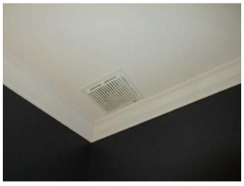
I was not able to turn on the exhaust fan of the washroom at the ground floor of the house. Fixing the exhaust fan is recommended.
