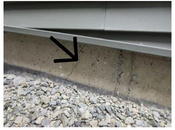
A crack was observed on the foundation wall on the south side of the house. It was 2 mm wide crack. Every crack or opening in the foundation wall is a potential source for moisture entry. The crack needs to be monitor for any changes contacting a qualified contractor for more action.
