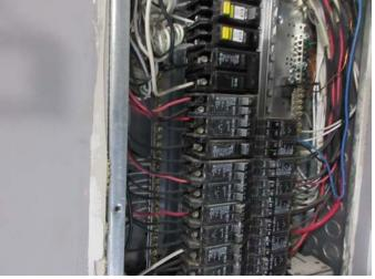
The electrical panel was 125 Amp and the main breaker was 125 Amp. The main panel was located in the north side of garage and professionally was installed. The wire type of the house was copper. It shows no burnt, damaged, or corroded wires. Breakers were labelled. Appropriate circuit breakers and sized wires were used for specific circuits (i.e. 40 amp for the range, 30 amp for the dryer, and 15 amp for general circuitry).
