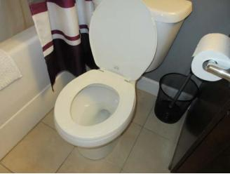
All toilets were tested at the house. The toilets and flushing of the house were functional at the time of this home inspection. No cracks or leaks to the flush tanks or toilets. No movement of toilet. The bowl was secure and was functioning with no deficiency at the time of this home inspection.
