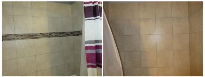
The master bathroom and main bathroom shower wall tiles and grout looks prefect with no deficiency at the time of this home inspection. The grout serving the shower tiles showed no deficiency at the time of this home inspection. Periodic sealing the connection point of the tile and the tub is necessary to prevent water penetration.
