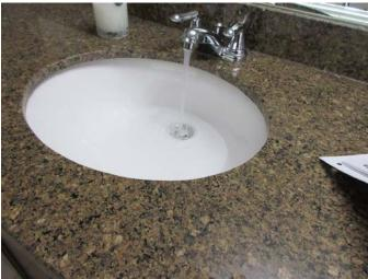
The water clogged was noted on the left basin sewage pipe at the master bathroom of the second floor and basement bathroom as well. The water was discharging slowly. Fixing the water clogged and the sewage pipe is recommended.
