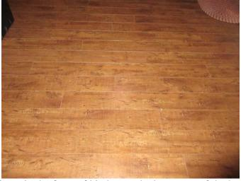
The floor coverage was laminate in the front of kitchen at the basement of the house. Minor bubbling laminate flooring was noted. Fixing the floor laminate is recommended.
