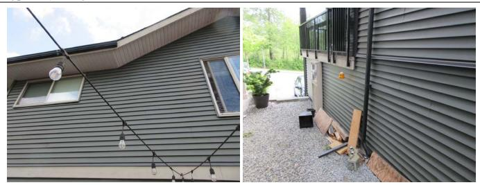
The house exterior wall had vinyl siding. The vinyl siding was functional with no deficiency at the time of this home inspection.
