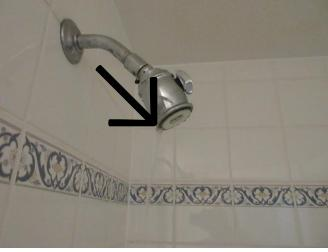
The water pressure looks low for the shower. The water leakage was observed on the faucet's spout at the master bathroom. The water leakage was noted on the shower head of master bathroom. Fixing the shower water leakage is recommended.
