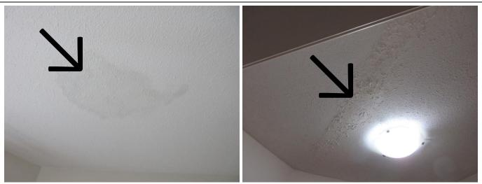
The old water leakage stain and damaged point was observed on the ceiling of the bedroom and corridor. The moisture stain and damage point was dry at the time of this home inspection. The moisture stain need to be monitored for any changes contacting a qualified contractor for more action as recommended.
