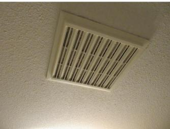
There were electrical exhaust fans in the bathroom and the washroom of the house. The exhaust fan in the master bathroom and main bathroom were functional at the time of this home inspection. The electrical exhaust fans grill was dirty and clogged with dust in the house. I recommend cleaning the grill of the fan for better functionality. The exhaust fan drill was loose in the master bathroom. Fixing the grill is recommended.
