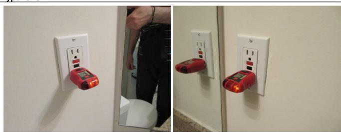
There were GFCI type outlet in bathrooms and in the washroom of the house. GFCI outlets were tested and appeared to be in serviceable condition on the day of this home inspection.
