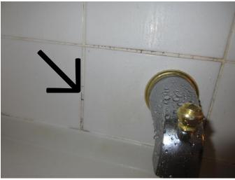
The wall tile grout was missed at the master bathroom of the house. The grout serving the shower tiles needs maintenance to prevent water entering the wall. Fixing the missed grout and periodic sealing is recommended.
