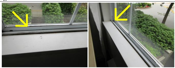
The dark stain and black spots were noted on the windows of master bedroom at the second floor unit. The black spots are suspicious and likely mold. Maybe mold or maybe not mold. Removing the minor black stain is recommended.
