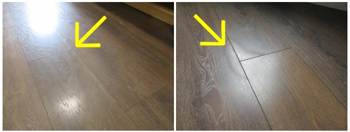
The house floor coverage was laminate. Minor buckling and lifting laminate flooring was noted at the second floor of the house. Fixing the floor laminate is recommended.
