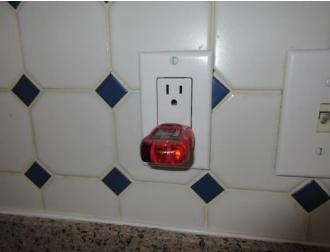
There were no GFCI type outlet in kitchen of the house. The regular outlet was installed in the kitchen of the house. It is safety concern. The outlet needs to be GFCI type in the kitchen to protect users from any electrical shock and unsafe situation. Ground Fault Circuit Interrupter (GFCI) outlets are recommended for installation at kitchen outlets.
