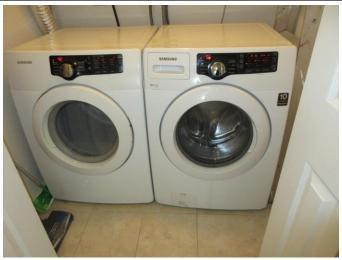
The washing machine and dryer were tested in the laundry room. There was no water leakage for washing machine. The washer and dryer were both functioning at the time of this home inspection.
