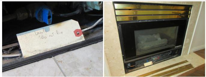
The house had gas fireplace type. The safe note was observed on the fireplace. I was not able to turn on the fireplace for this, I could not perform a reasonable inspection. The fireplace had the smoke glass. Cleaning the fireplace glass and remove the smoke is recommended.
