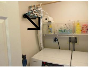
The dryer had foil duct which is not recommended for the dryer. This is a safety concern. It is a potential fire hazard. The hard metal or aluminume type duct only is accepted and recommended for dryer. I recommend installing the hard metal or aluminum duct for the dryer.
